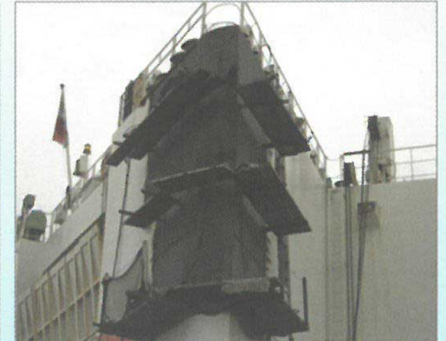
• Hull plate renewal
